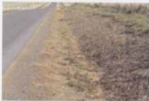
Fig. 1 Road verge and table drain sprayed twice in clear vegetation. Storm water runoff can flush pollutants from road surface directly via drains into our creeks without first filtering through a grassy filter strip.
