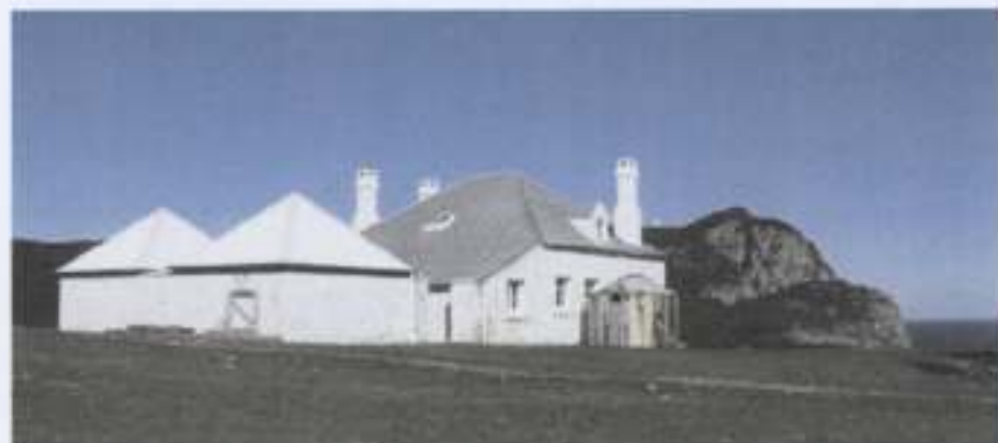
The lighthouse superintendent's house is now a museum open to the public.
